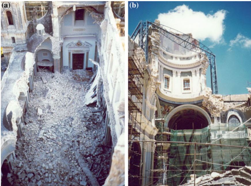
Fig. 2.68 a The interior of the church after collapse; b The collapsed dome
