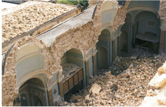
Fig. 2.72 The massively thick concrete of the arches and small domes
