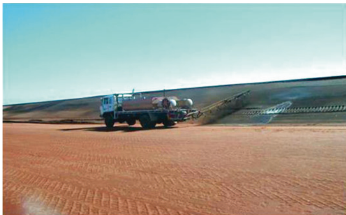
Fig. 9 Bitumen emulsion being sprayed to reduce dust from embankment walls. Adapted from Alcoa World Alumina Australia, March 07.
