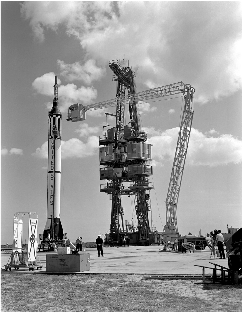
The “cherry picker” (more correctly the “mobile aerial tower”) acted as an emergency escape route for an astronaut in peril. (Photo: NASA)
