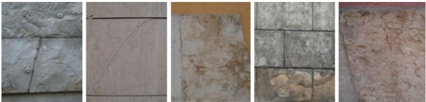
Fig. 2.5 Loss-of-integrity defects in natural stone claddings (from left to the right ): fracture, cracking, erosion, exfoliation and alveolarization of stone plate
