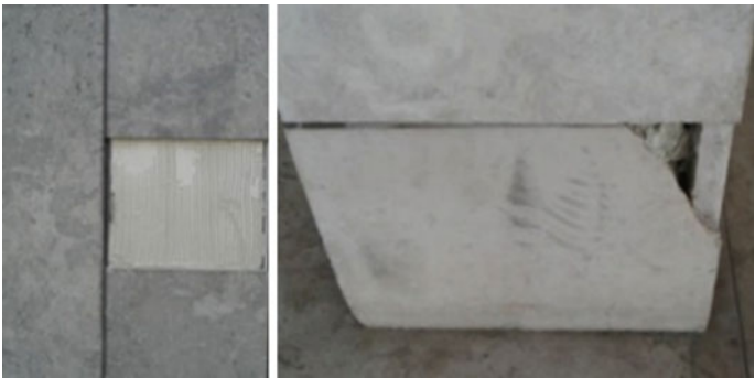
Fig. 2.4 Bond-to-substrate defects in natural stone claddings (from left to the right ): loss of an element in the stone cladding and partial loss of stone material
