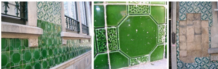
Fig. 2.19 Case study that illustrates the end of the service life of ceramic claddings (with a severity of degradation around 20 %) (data sourced from Bordalo 2008)
