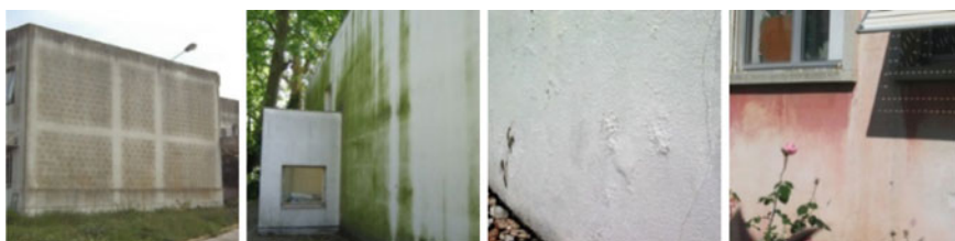
Fig. 2.6 Visual or surface degradation defects in rendered façades (from left to the right ): thermophoresis, biological growth, efflorescence, colour change (data sourced from Gaspar 2009)
