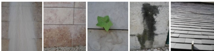
Fig. 2.2 Visual or surface degradation defects in natural stone claddings (from left to the right ): efflorescence, localized stains (rising damp), parasitic vegetation, biological growth and flatness deficiencies
