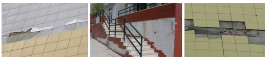
Fig. 2.15 Detachment defects in ceramic tiling systems: debonding ( left ) and detachment of ceramic tiles (data sourced from Bordalo 2008)
