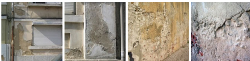
Fig. 2.8 Loss of adhesion or cohesion in rendered façades (from the left to the right ): detachment, pulverulence, arenization, erosion (data sourced from Gaspar 2009)
