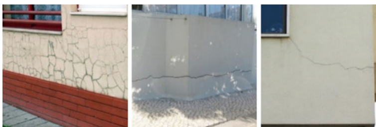
Fig. 2.7 Cracking defects: mapped cracking in rendered façades ( left ) and oriented cracking ( right ) (data sourced from Gaspar 2009)
