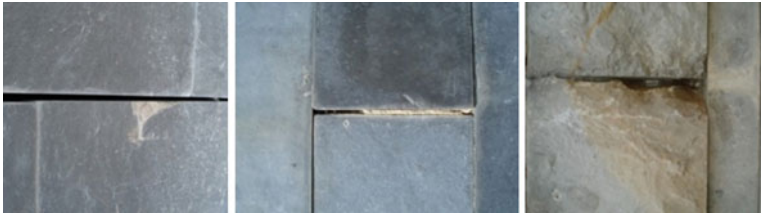
Fig. 2.3 Joint defects (from left to the right ): lack of linearity between the joints of stone plates, material loss—open joint and scaling of stone near the joints
