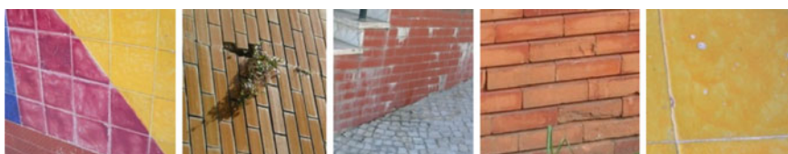
Fig. 2.12 Visual or surface degradation defects in ceramic tiling systems (from left to the right ): localized colour change, parasitic vegetation, efflorescence, crushing or scaling of the borders and small superficial craters (data sourced from Bordalo 2008)
