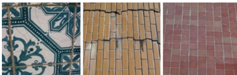
Fig. 2.13 Cracking defects in ceramic tiling systems (from left to the right ): cracked glazing, markedly orientated cracking and with no predominant direction (data sourced from Bordalo 2008)
