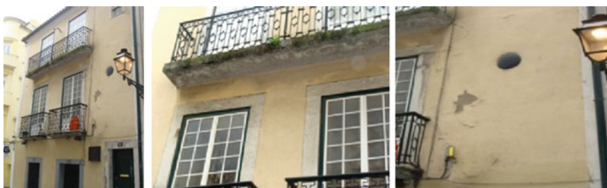
Fig. 2.18 Case study that illustrates the end of the service life of painted surfaces (with a severity of degradation around 20 %) (data sourced from Chai et al. 2014 )
