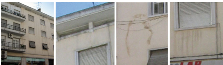
Fig. 2.17 Case study that illustrates the end of the service life of rendered façades (with a severity of degradation around 20 %) (data sourced from Gaspar 2009 )
