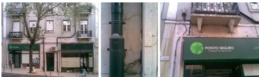
Fig. 2.16 Case study that illustrates the end of the service life of stone claddings (with a severity of degradation around 20 %) (data sourced from Silva 2009 )
