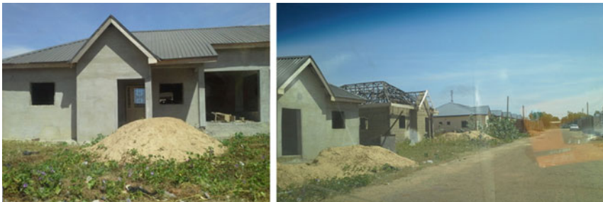
Typical two bedroom low income public housing scheme under construction in Sokoto, Nigeria
