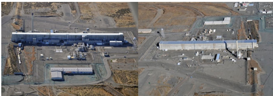
Fig. 2.7 PUREX Plant in Hanford, Washington [27]. The PUREX “canyon” was over 1000 feet long, 60 feet wide, and 100 feet high [32]
