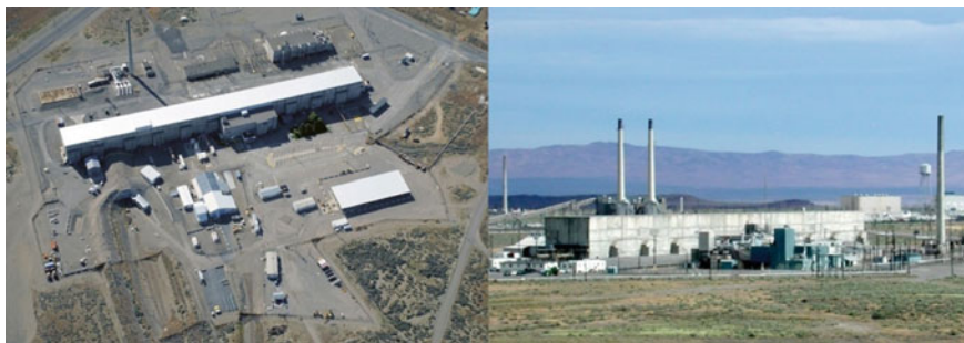
Fig. 2.4 T Plant ( left ) and U Plant ( right ) in Hanford, Washington [27]. “Canyons” such as these could be larger than 800 feet long, 85 feet wide, and 100 feet high
