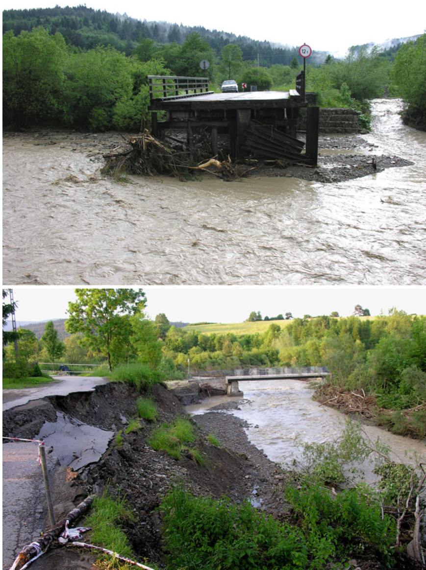
Fig. 2 Damage to infrastructure caused by the 80-year flood of June 2010 on the Biała River. A significant increase in forest cover in the catchment after World War II and widespread in-channel gravel mining conducted in the past decades resulted in sediment starvation of the river and thus the flood action was mainly directed on erosion of the channel boundaries
