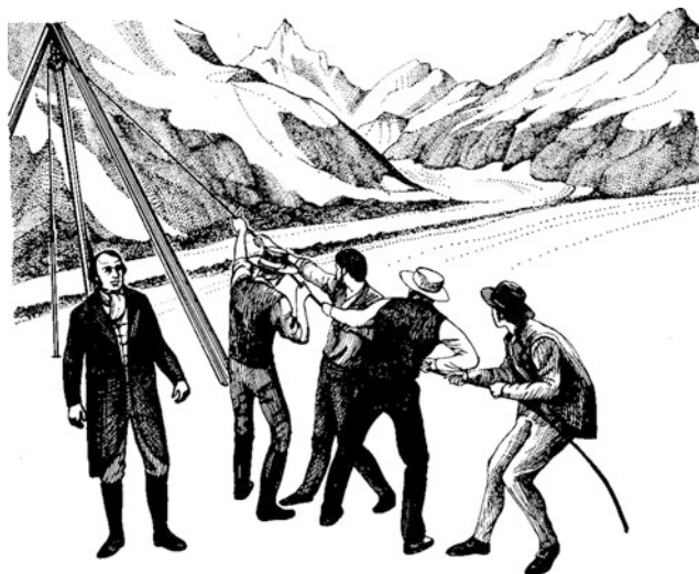
Fig. 2.2 Cable tool used by L. Agassiz in 1842 (Clarke 1987)
