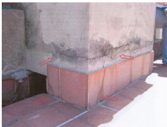
Fig. 19 Cracks on the mortar indicating the displacement of the waterproofing blanket (Nov 2005 —Cerne Engenharia)
