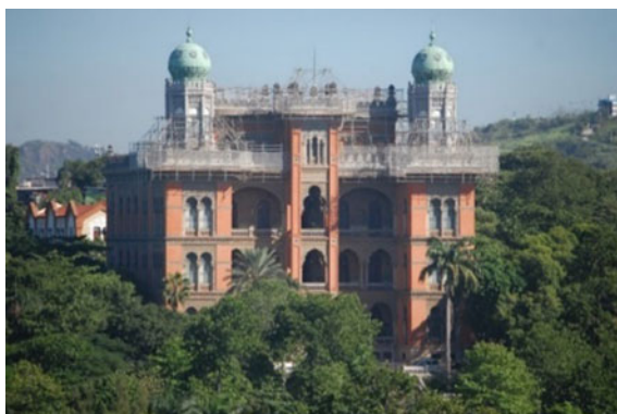
Fig. 23 Suspended scaffolds covering the front of the Pavilhão Mourisco's terraces, on the intervention's first phase (Apr 2014)
