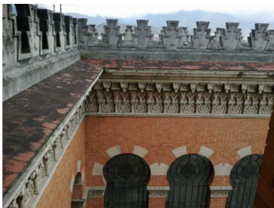
Fig. 22 Black crust on the external ceramic tiles (May 2014)
