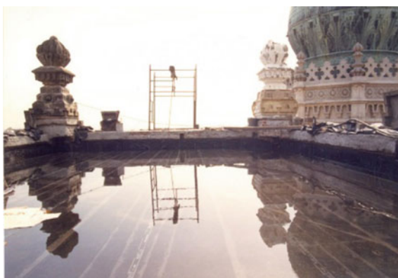
Fig. 13 Testing the new butyl rubber blanket with a layer of water over it for 72 h —seventh-floor terrace (1990)
