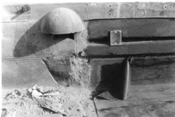
Fig. 10 Separation from the untreated surface ( on the left ) and the butyl rubber blanket ( on the right ) on the fifth floor (1988)
