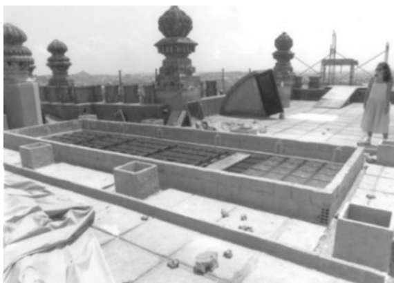
Fig. 14 Construction of the shelter dome for the skylight on the seventh-floor terrace (1990)
