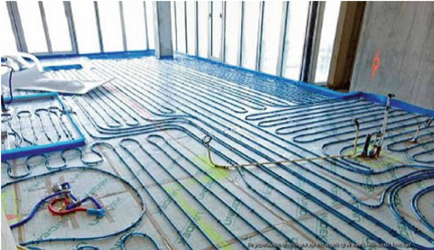
Fig. 2.5 Under-floor heating/cooling of the apartments of De Rotterdam
