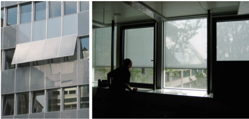
Fig. 2.47 Automated exterior solar control screens applied as a facade retrofit ( revitalisierung ) to the Haupthaus KfW building in Frankfurt ( left ) and interior view with screens deployed ( right )
