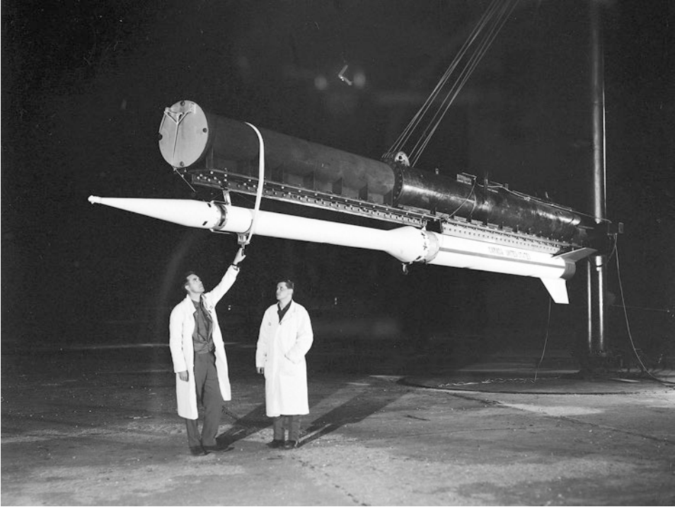
Fig. 2.11 DRB engineers inspect a BBIV on its launch rail c.1963
