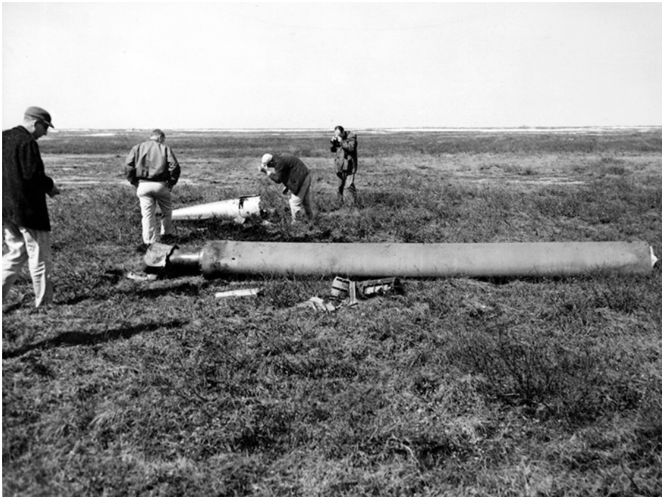
Fig. 2.13 DRB technicians recover the remains of a Black Brant IV rocket somewhere north-east of the Churchill Research Range, July 1964
