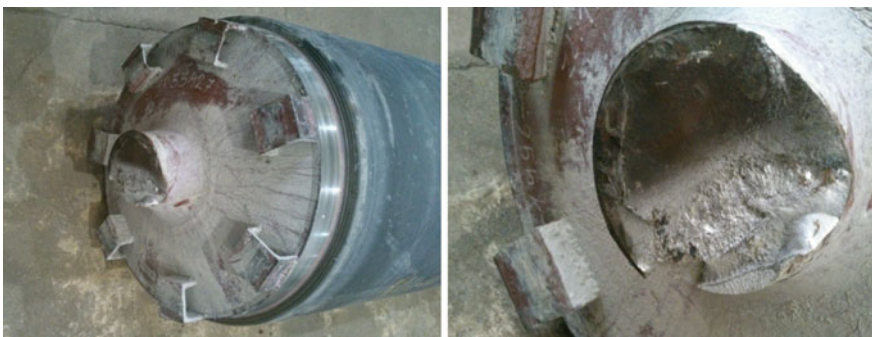
Fig. 2.24 Examples of damages—fracture of the drive drum of a bucket-wheel excavator's belt conveyor
