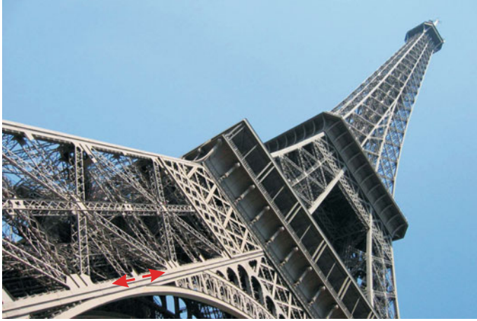
Fig. 2.39 The effect of a point load on the top of the Eiffel tower on a truss element depends on how sensitive the top is to a unit spread of the truss element
