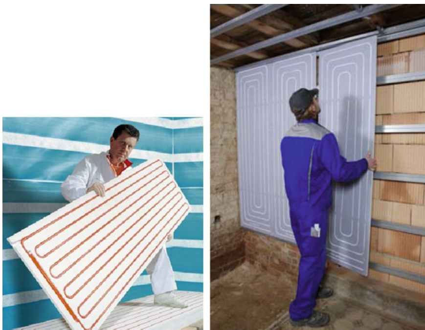
Fig. 2.22 Wall radiator made using the dry technology [39, 40]
