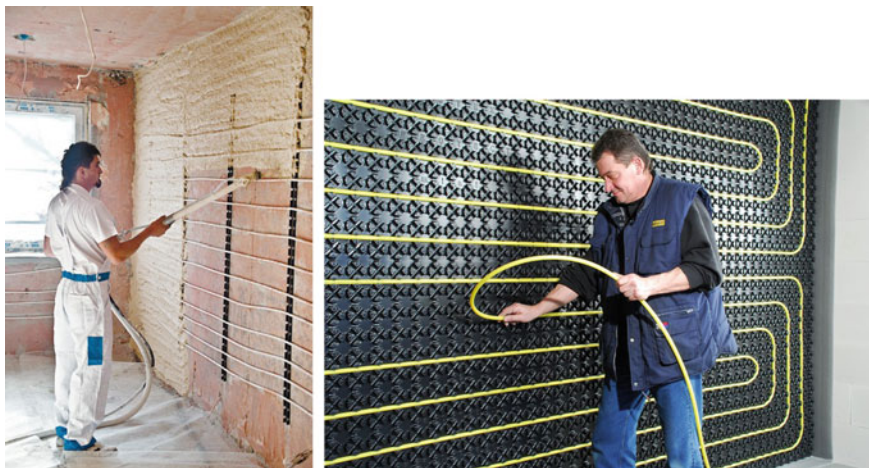
Fig. 2.21 Wall radiator made using the wet technology [37, 38]
