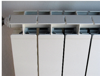
Figure 2.17: Details of a domestic radiator. In order to increase the heat flow rate, the metal-to-air contact area is increased by the flat design, introducing sections and columns, and adding convector fins.
