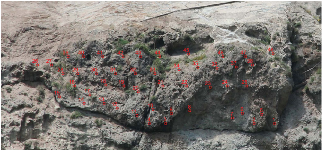
Fig. 31 Positioning of the the 48 installed dowels
