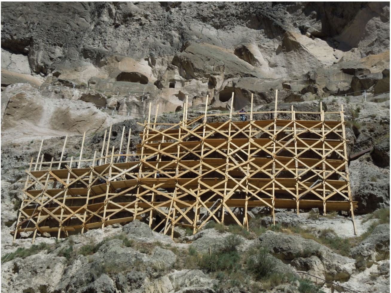
Fig. 30 The wood scaffolding realised in Vardzia
