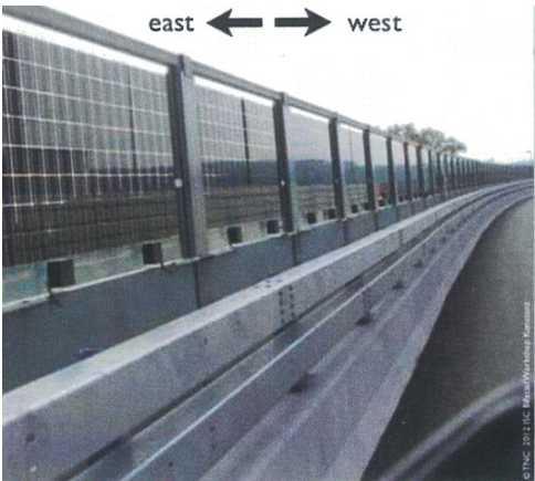
Fig. 6 Swiss highway with vertically installed bifacial modules (Source: 8; TNC)
