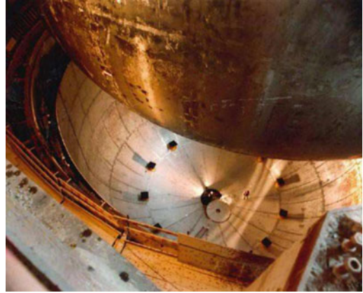
Fig. 2.16 Introduction of the main vessel into the safety vessel. The chocks between the two vessels are visible
