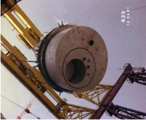
Fig. 2.26 Lifting the two rotating plugs
