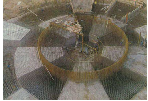
Fig. 2.2 View of the base-mat reinforcement steel in progress on January 20, 1977
