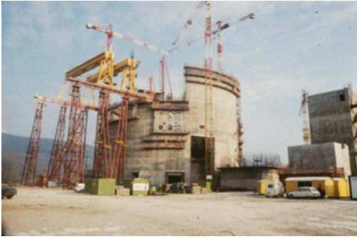
Fig. 2.8 The reactor block construction continues with the transfer gantries
