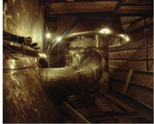
Fig. 2.28 Assembling the pump/diagrid link
