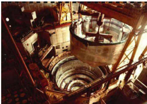
Fig. 2.20 Introduction of the third package into the main vessel
