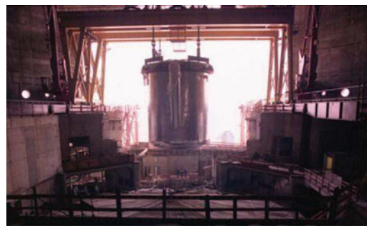
Fig. 2.30 The storage drum arrival upright its pit
