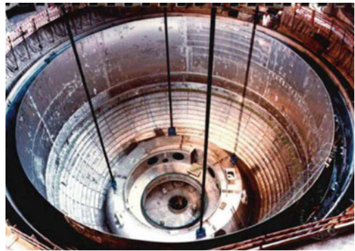
Fig. 2.17 View of the second package on its chocks in the safety vessel
