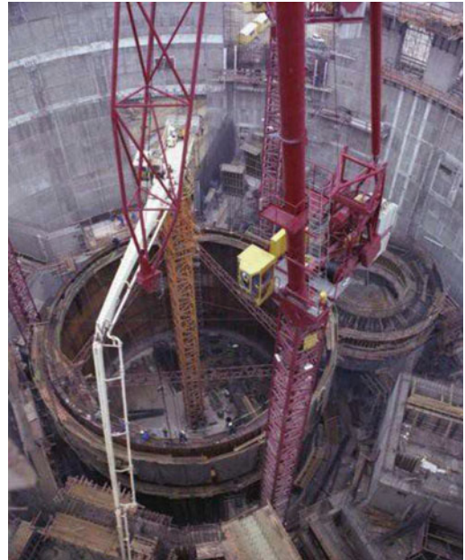
Fig. 2.7 Reactor pit and storage drum pit construction
