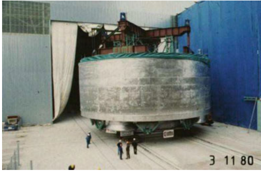
Fig. 2.19 The third package getting out from the workshop, on rails
