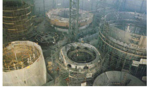
Fig. 2.12 Fabrication in simultaneous activities of several packages in the on-site workshop
