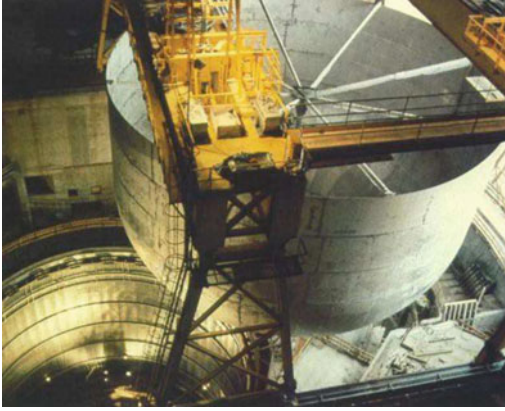
Fig. 2.14 Arrival of the first package (safety vessel) in the reactor block
