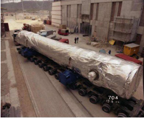
Fig. 2.4 On site arrival of a steam generator
