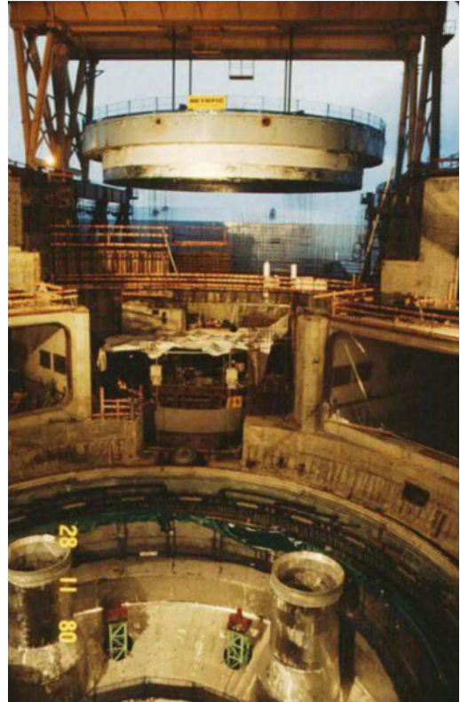
Fig. 2.21 Arrival of the reactor slab
