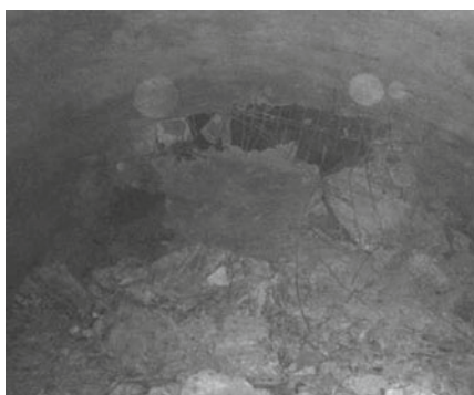
(a) Cracking of primary support
