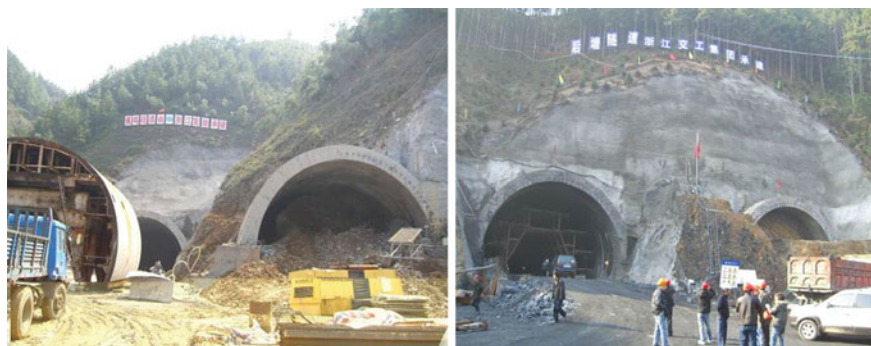
Fig. 2.28 Field photos for excavation of small-clearance tunnels using pilot tunnel method
