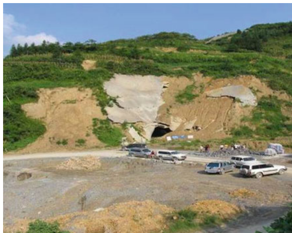
Fig. 2.7 Surrounding rock failure caused by delayed supporting
