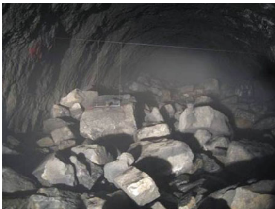
Fig. 2.6 Collapse of a carven after excavation
