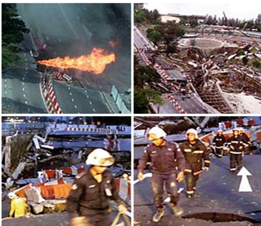
Fig. 2.17 Continuous collapse of street pavement caused by underground works (mutual impact)
