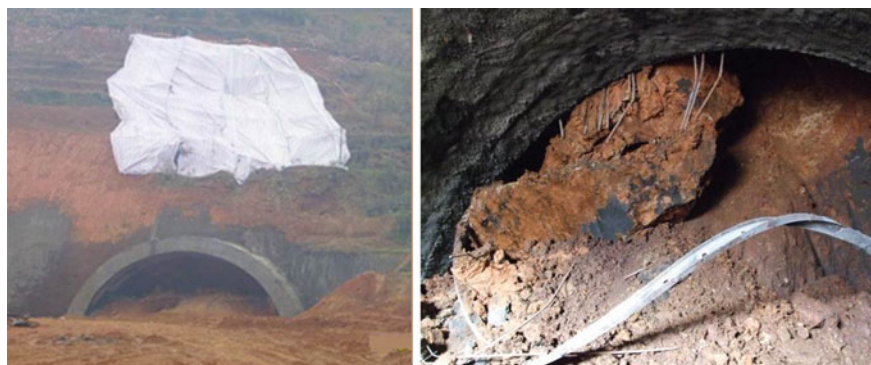
Fig. 2.13 Tunnel collapse accident caused by supporting design parameters according to design code
