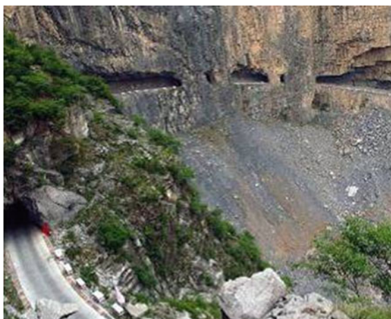
Fig. 2.5 The surrounding rock is able to self-stabilize after excavation
