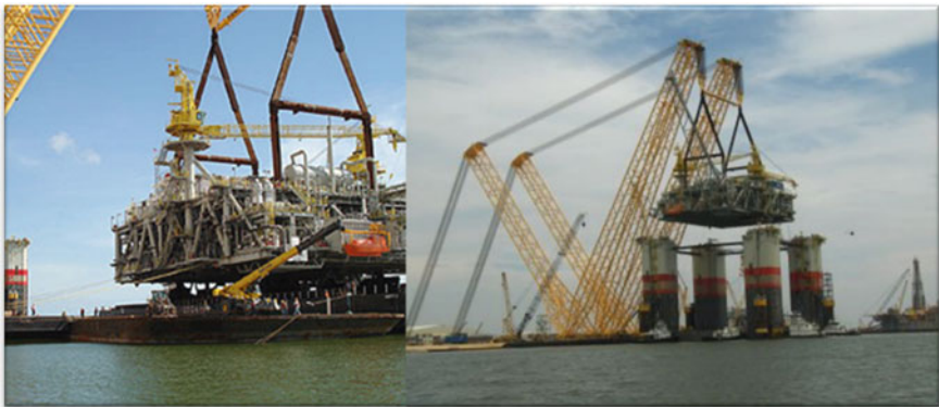
Fig. 2.31 The platform integration of Chevron Blind Faith DDS. The topsides is an integrated topsides. HLD (Heavy Lifting Device) lifted the integrated topsides from the transportation barge ( left ) and put on the hull ( right ) (courtesy of Rigzone and KOS)
