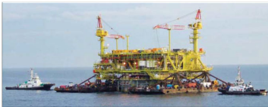
Fig. 2.58 Murphy's Kikeh truss spar platform integration offshore Malaysia in November, 2006 was the first open water catamaran floatover operation and was successful (courtesy of Technip)
