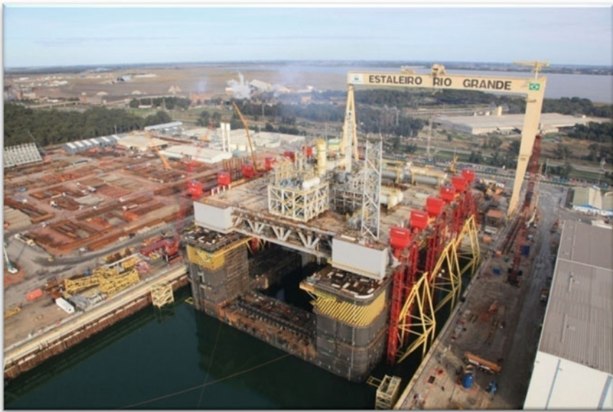
Fig. 2.42 The topsides and the hull were aligned and ready for mating (courtesy of Petrobras)
