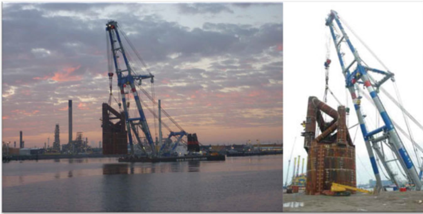
Fig. 2.13 Suction bucket with leg stiffening frame on the top is lifted by Matador 3 and put in position to be connected to the platform leg (courtesy of ©Heerema Fabrication Group)
