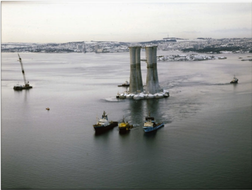
Fig. 2.26 Condeep Statfjord B was towed to the integration site at Yrkje Fjord in Vindafjord. (Courtesy of Statoil)
