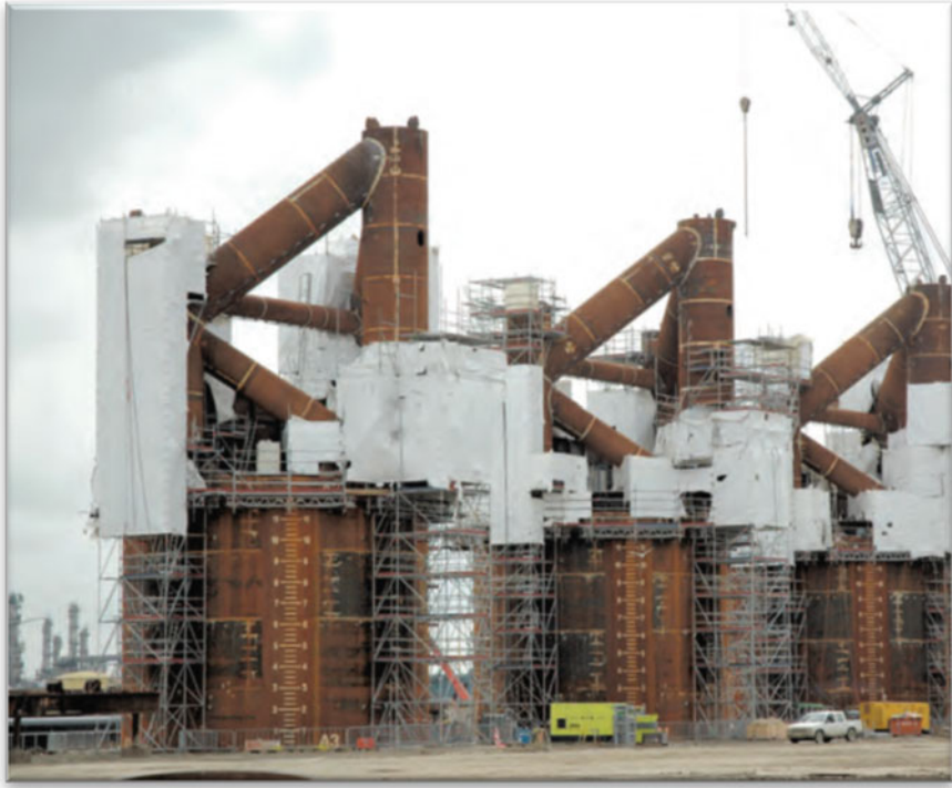
Fig. 2.11 For each suction pile, the leg-stiffening frame was already welded to it and the assembly was ready to be connected to the platform leg (courtesy of Han Heilig, publisher of Offshore Holland, the Netherlands)
