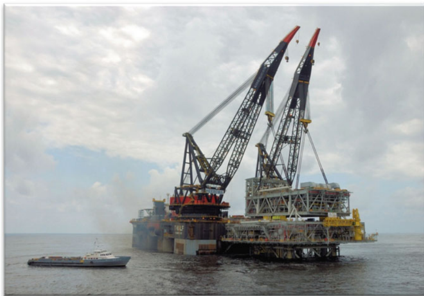
Fig. 2.51 The Center Module was lifted and put on the MSF of the Chevron TOL (Tombua Landana) compliant tower platform in offshore Angola (courtesy of Chevron)
