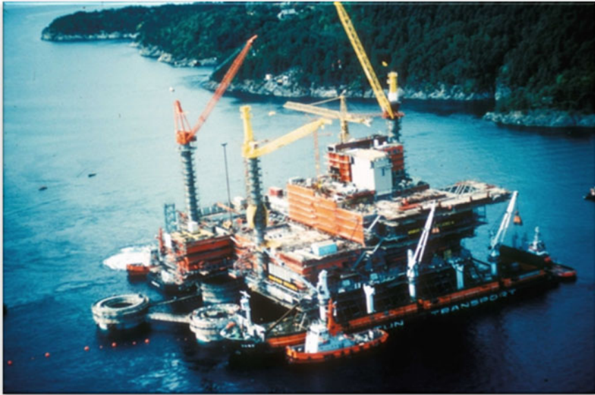
Fig. 2.32 Mating operation of Statfjord A. The topsides was not an integrated topsides, a few modules were installed on the MSF which is carried by two tankers and then floated over the shafts of the base which was only a few meters above the water surface (courtesy of Norwegian Petroleum Museum)
