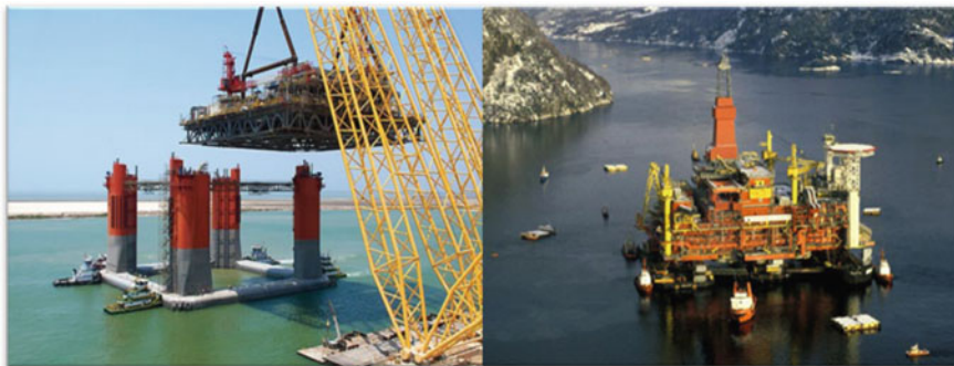
Fig. 2.25 The integration site should be carefully selected for successful mating operation. On the left is the topsides installation by heavy lifting for WHO DAT topsides. On the right , it shows the topsides of Statfjord B being carried out on barges near the mating site ready for floatover (courtesy of KOS and StatOil)
