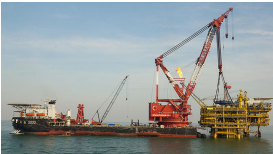
Fig. 2.47 The topsides of a fixed platform was installed by a crane barge (courtesy of CNOOC)
