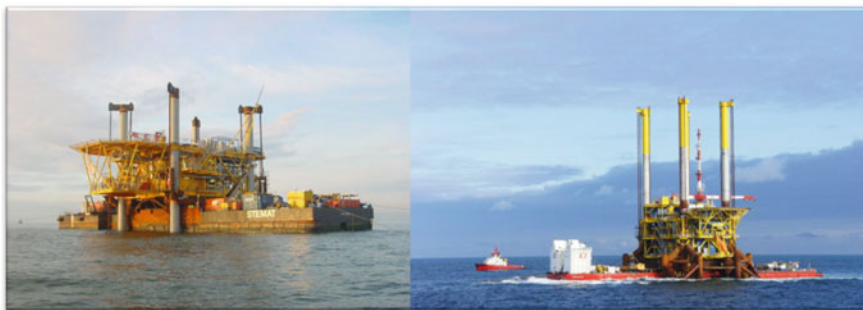
Fig. 2.8 SIP II concept platforms: on the left is Calder SIP II platform in 30 m water depth in Irish Sea, UKCS; on the right is F3-FA SIP II platform in 40 m water depth near Dogger Bank in the North Sea (courtesy of SPT Offshore)
