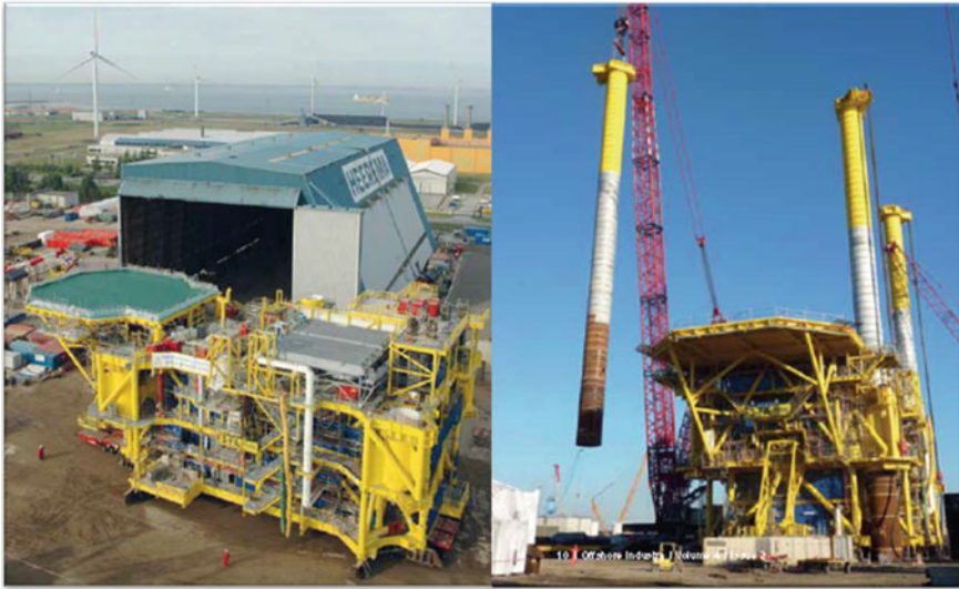
Fig. 2.10 On the left , the fabrication of the 4000 t topsides is completed and moved out from the fabrication hall and ready for the leg installation; on the right shown the installation of the legs by the yard crawler cranes (courtesy of Centrica Energy)
