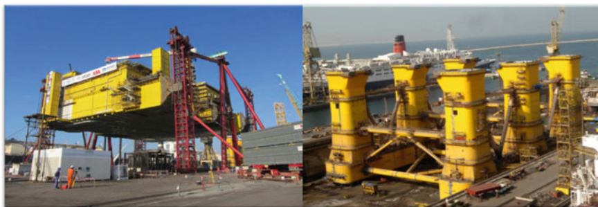
Fig. 2.44 Both of the topsides and the hull were built in the drydock of the Drydocks World yard at Dubai, the topsides was fabricated in the drydock (courtesy of Drydocks World and ALE)
