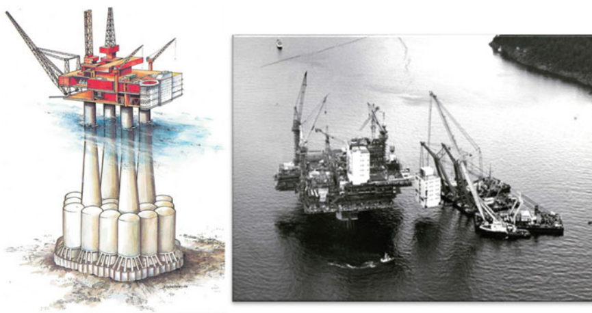
Fig. 2.28 Condeep Statfjord A and the installation of topsides modules (courtesy of Statoil and Norwegian Petroleum Museum)
