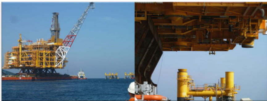
Fig. 2.54 SHWE platform integration in Bay of Bengal, Myanmar. The weight of the topsides is 26,000 Mt carried by the COOEC barge HYSY 229 (courtesy of Dockwise)
