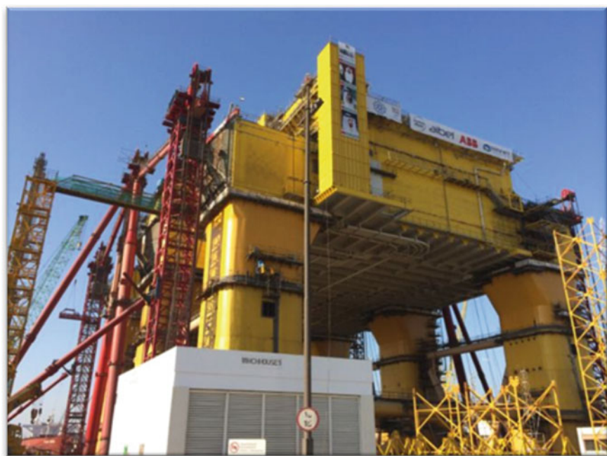
Fig. 2.45 The topsides of the Dolwin Beta was lowered on the columns of the semisubmersible look-like GBS hull, the ALE's gantry system can be seen clearly (courtesy of Drydocks World and ALE)
