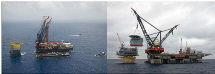
Fig. 2.50 In early 2009 HMC installed the integrated topsides of the Perdido with a 9773 ton single lift by their SSCV Thialf, a record for the US part of the GOM. The living quarter was then put on the topsides. It took two weeks to complete the installation (courtesy of HMC and Shell)
