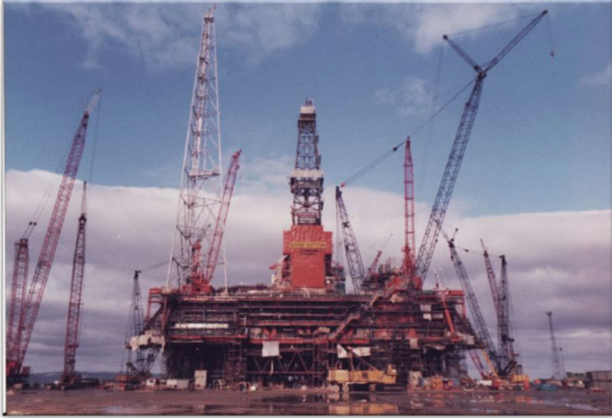
Fig. 2.37 The topsides of Conoco (UK) Ltd's Hutton TLP was under construction at Ardersier Yard (courtesy of Oilrig-Photos)
