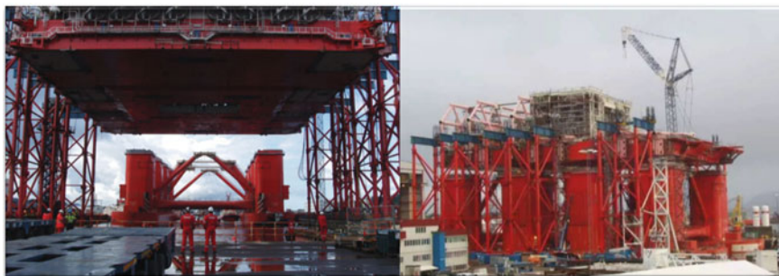
Fig. 2.43 Aker H6-e semisubmersible drilling rig was integrated at the drydock of Aker Stord yard (courtesy of Aker Solutions)
