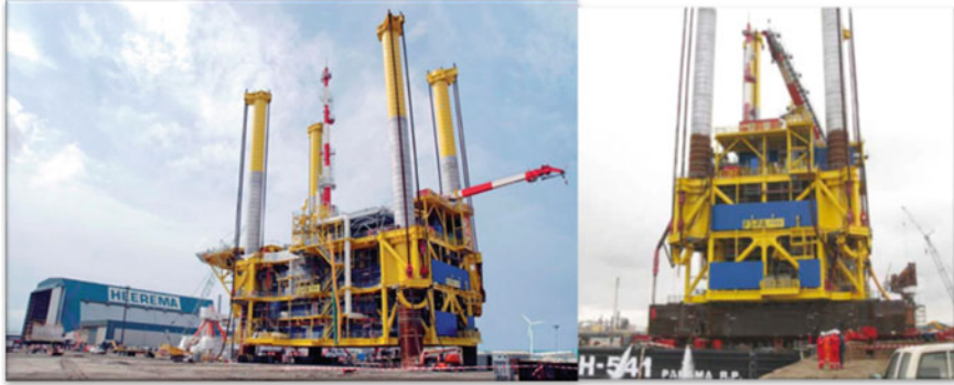
Fig. 2.12 Loadout of F3-FA topsides. On the left , it shows the topsides was being loaded out to the transportation barge at the fabrication yard. On the right the topsides was first moved on board Heerema barge H-541 and then positioned on Boa Barge 35 (courtesy of ©Heerema Fabrication Group)
