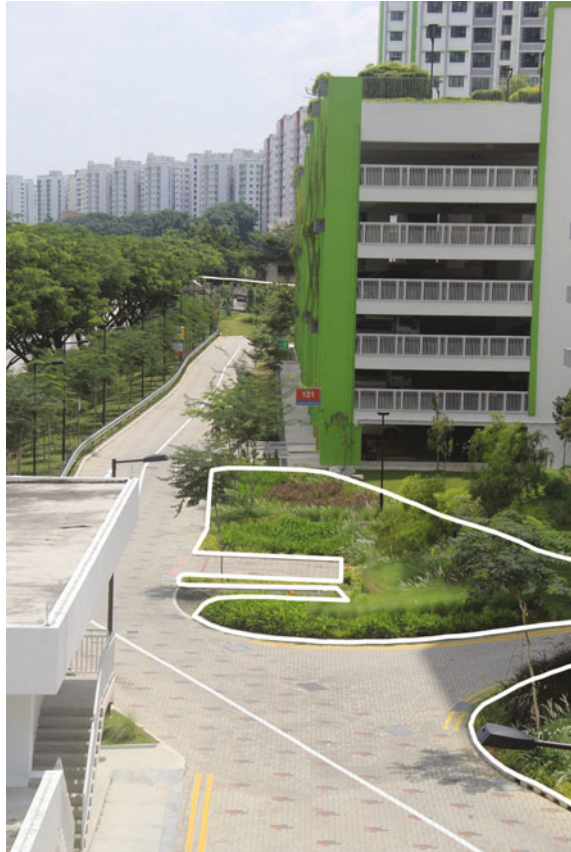
Fig. 2.3 A rain garden designed to treat stormwater runoff from the service road of a residential estate in Singapore (marked in white lines ). Note however that the treatment is highly localized; and runoff from upstream and downstream in the same road, as well as runoff from other paved areas in this precinct are not treated. Overall net benefits for stormwater management at the precinct scale can be questioned
