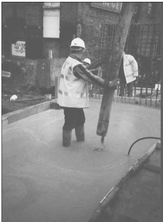
Fig. 2.18 Placement of SCC by pump tremie on site, demonstrating the flowable nature of the material (Mott MacDonald Ltd). Reprinted from Ref. [65], with permission from ICE Publishing
