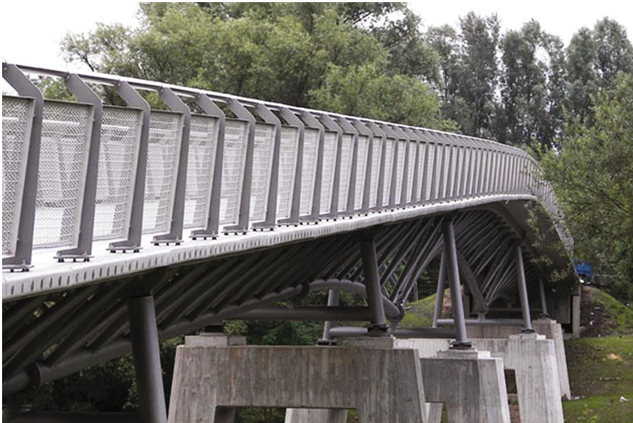
Fig. 2. Gärtnerplatz bridge in Kassel as the first UHPC construction in Germany; Photo: University of Kassel
