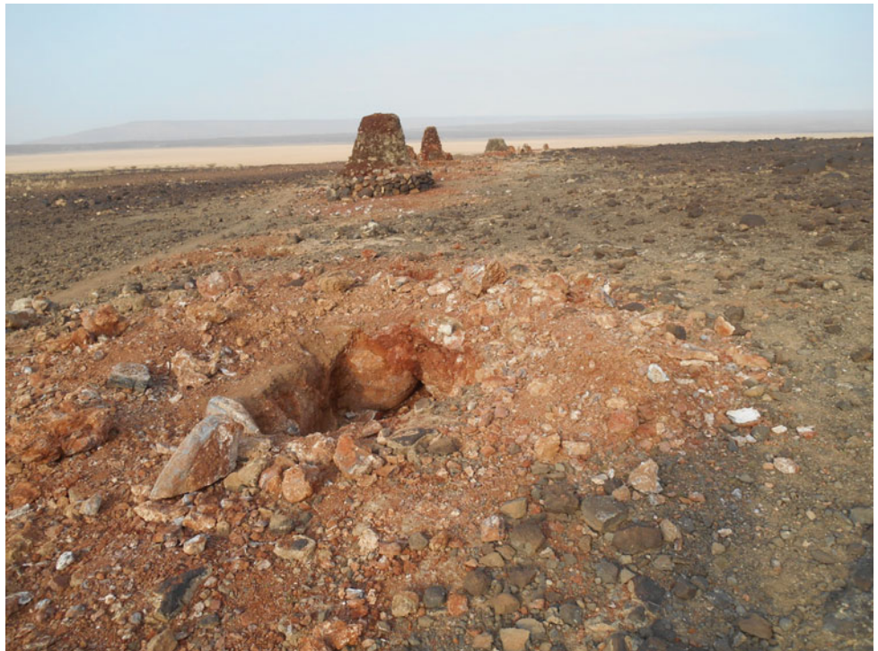
Fig. 2.13 In central Afar, along an open fissure cutting through the Stratoid series, from which the steam surge, producing clay alteration products as well as carbonate and silica deposits, a set of water condensers is being built for drinking water collection and bathing developments ( Photo J. Varet 2015 )
