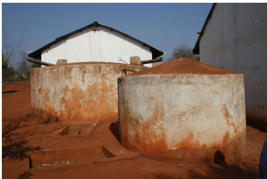
Fig. 4 Roof catchment system with ferro-cement tanks. Photograph Josep de Trinchieria Gomez
