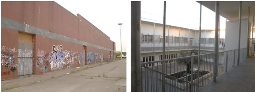
Fig. 2.13 Demalling of the former medium-size structure bearing the Esselunga sign in Pioltello (MI): Facade and internal courtyard
