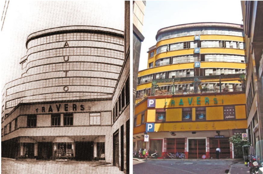
Fig. 2.3 Former garage Traversi, via Bagutta, Milan (1938 and 1986). Source http://www.lombardiabeniculturali.it
