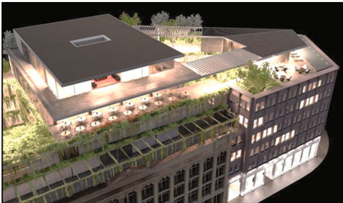
Fig. 2.8 The design for Palazzo Broggi (formerly Unicredit). Source http://www.piuarch.it
