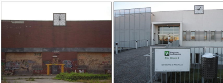
Fig. 2.12 Demalling of the former medium-size structure bearing the Esselunga sign in Pioltello (MI)
