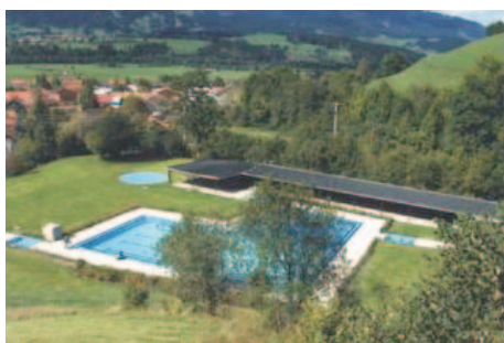
Fig. 4.3.10. Solar plant for an open air swimming pool (350 m 2 absorber surface), Germany (Allgäu).
