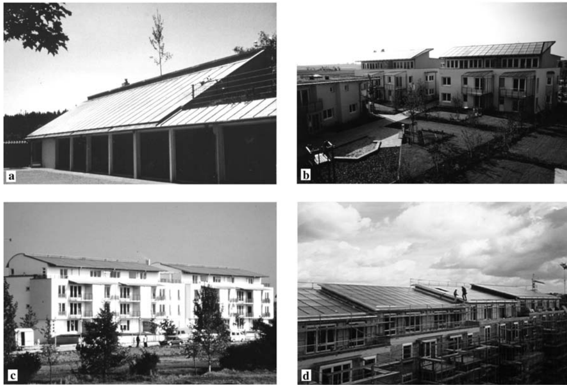
Fig. 4.3.20. (a) Collector field ( 115 \text{ m}^2 ) mounted on a garage in Ravensburg (No. 1 in Table 4.3.1). (b) 160 \text{ m}^2 roof integrated collector area in Köngen “Burgweg West” (No. 3 in Table 4.3.1). (c) Collector fields of multiple dwellings in Neckarsulm-Amorbach (No. 4 in Table 4.3.1). (d) Installation of the collector fields in Stuttgart-Burgholzhof (No. 10 in Table 4.3.1).
