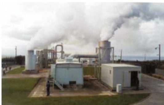
Fig. 8.48. Direct-intake, non-condensing single flash geothermal power plant at Pico Vermelho (São Miguel Island, Azores) exhausting steam to the atmosphere [04Lun2].
