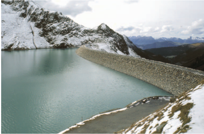
Fig. 2.3.13. Finstertal Rockfill dam, 1981, Austria. Crest length = 652 m, height = 149 m.
