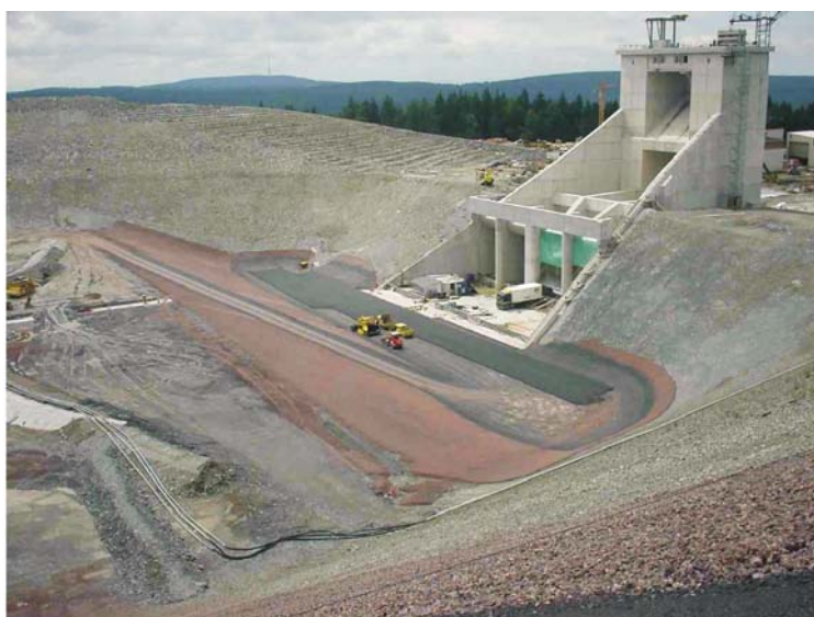
Fig. 2.6.6. Lateral intake structure arrangement in the dam (Goldisthal, Germany).
