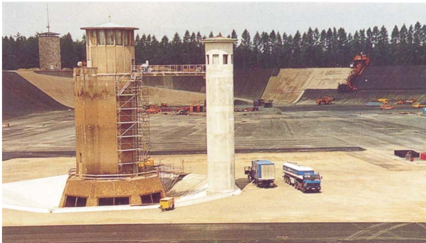
Fig. 2.6.7. Intake and access tower connected via catwalk (Rabenleite, Germany).
