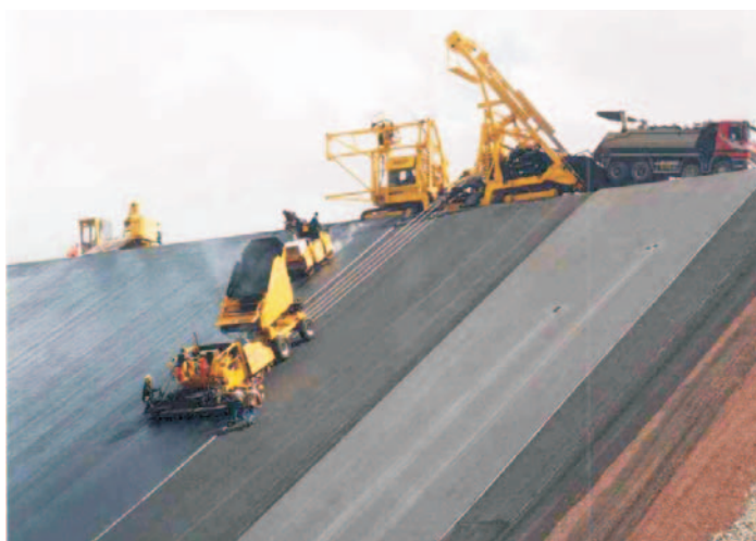
Fig. 2.6.5. Asphaltic sealing applied on a dam-slope.
