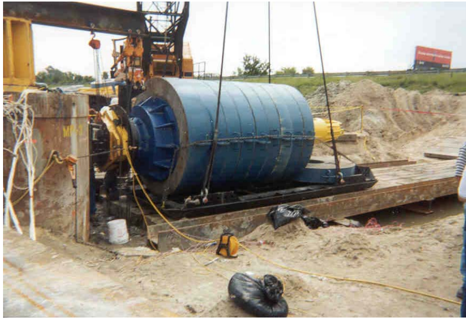
Figure 4. Photograph of static load sled being moved into position for load test.
