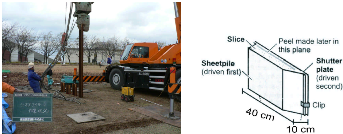
Figure 4. Photographs of sheet pile driving and a schematic diagram of the sampling system
