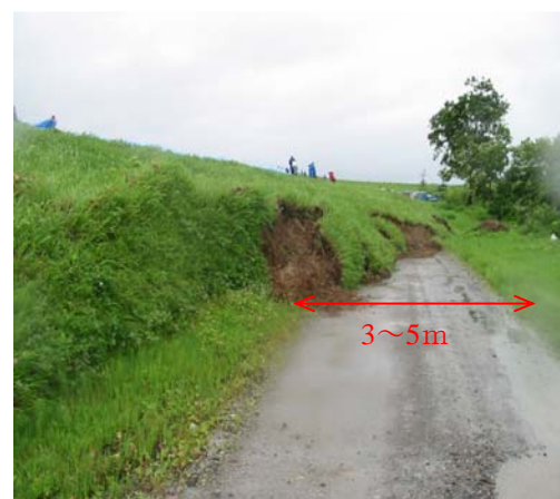
Figure 6. Flow of sediment on land side at Kimazuka
