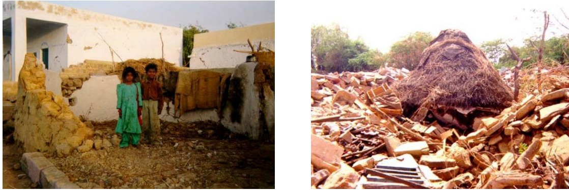
Figure 1: Typical Collapse of Adobe Buildings in the 2001 Bhuj Earthquake, Choudhary et al (2002)
