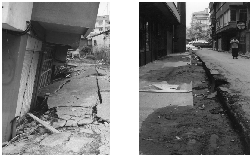
Figure 4. Building damage in the form of foundation bearing failure at soft sites
