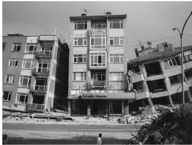
Figure 3. Building damage in the form of bearing system failures at stiff sites
