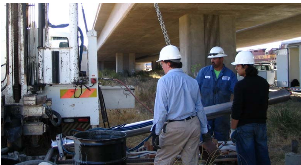
Figure 4. Lifting the DFSD off the transport cart, into vertical position prior to deployment.
