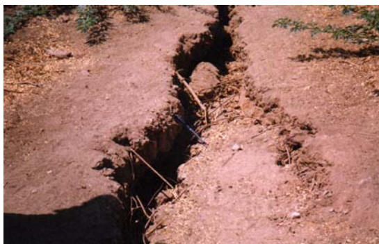
Figure 4. Longitudinal Crack along the length of Ratiya dam
