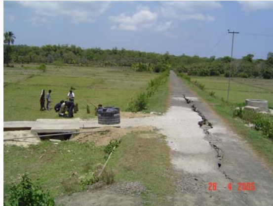
Figure 11 : Complete and close up View of Longitudinal crack along the rural embankment
