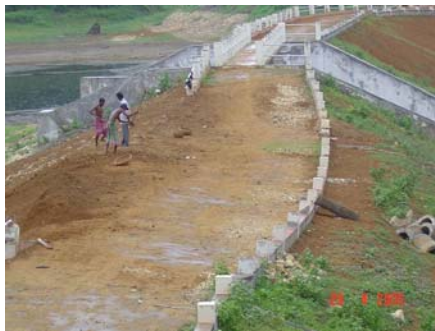
Figure 9: Loss of alignment of Vishnu Nalla Dam
