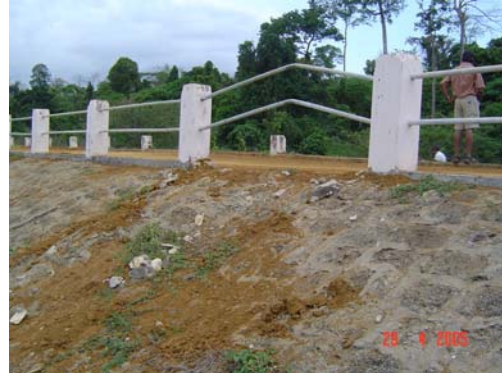
Figure 8 : Side rails and side slope of embankment dam still in distress
