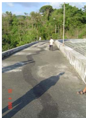
Figure 6: Longitudinal crack developed all along the length of rockfill dam
