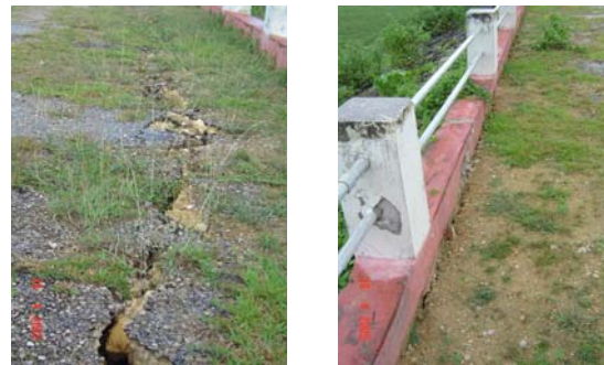
Figure 10: Longitudinal crack on the Vishnu Nalla earthen dam
