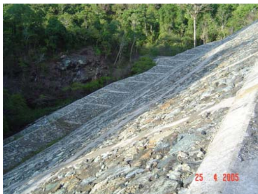
Figure 5 : Side slope of rockfill dam that experienced some disturbance
