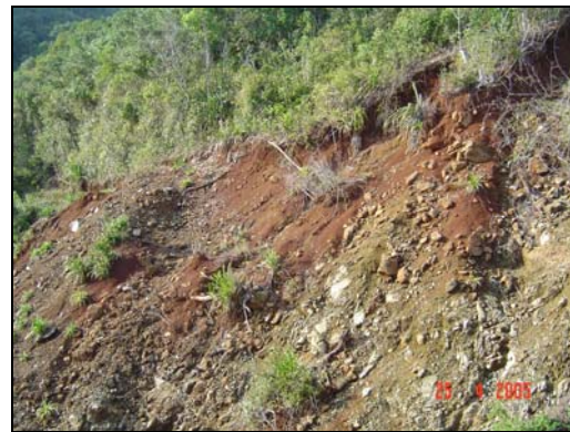
Figure 4 : Picturesque hill side slopes experienced slope failure
