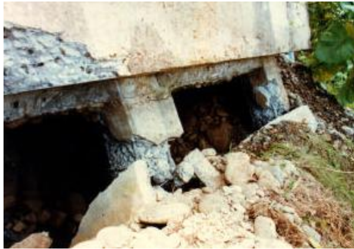
Figure 3. Preferential Damage to Front Batter Piles of Rio Banano Bridge during the 1991 Costa Rican Earthquake (after Priestly et al., 1991)
