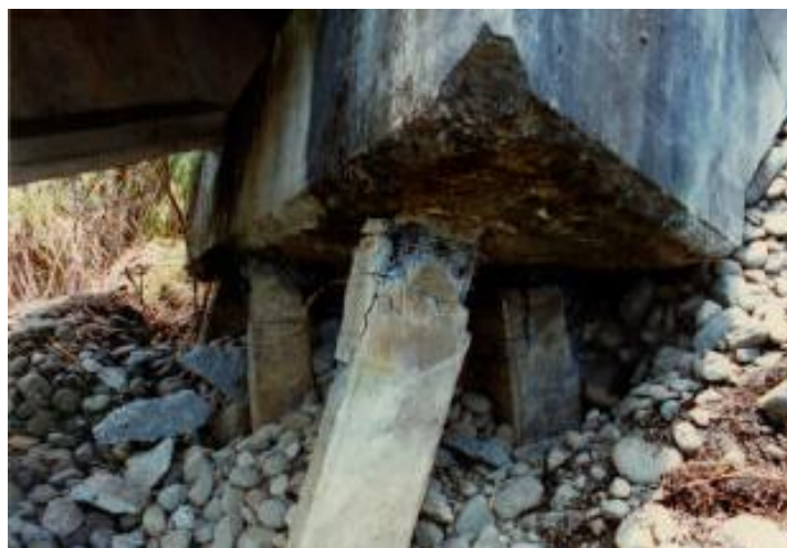
Figure 4. Failure of Rio Viscaya Bridge Piles during the Costa Rican Earthquake (after Priestly et al., 1991)
