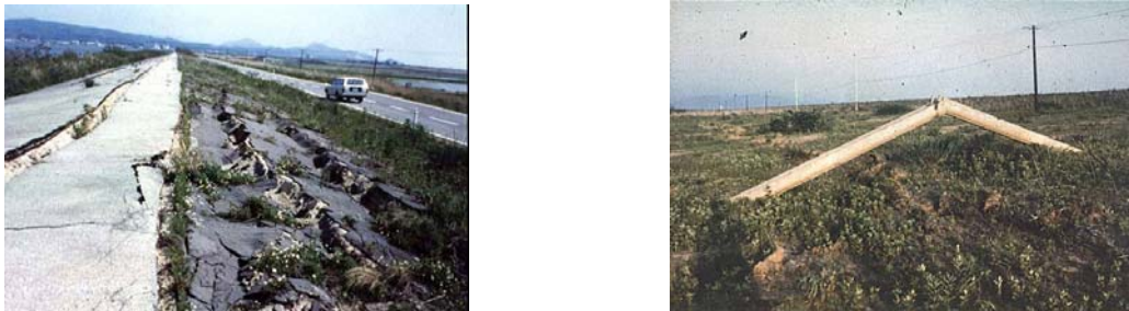
Figure 12. Longitudinal cracks and uplifted gutter seen at the Hachirogata dike in 1983
