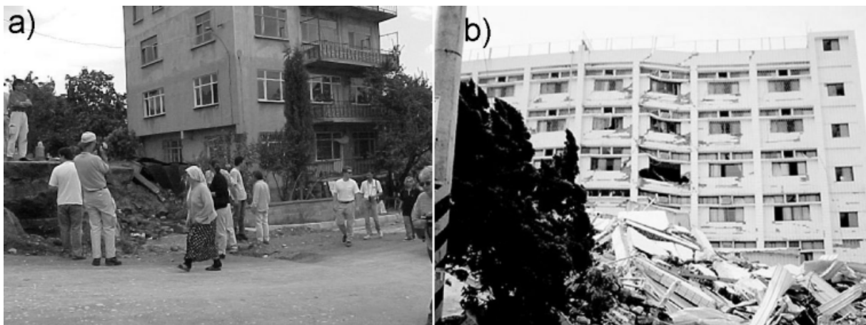
Figure 1. Dip-slip fault rupture near/through structures. a) Gölcük, Turkey, photograph by EERI; b) Wu-Feng, Taiwan, photograph by K.I. Kelson, EERI.
