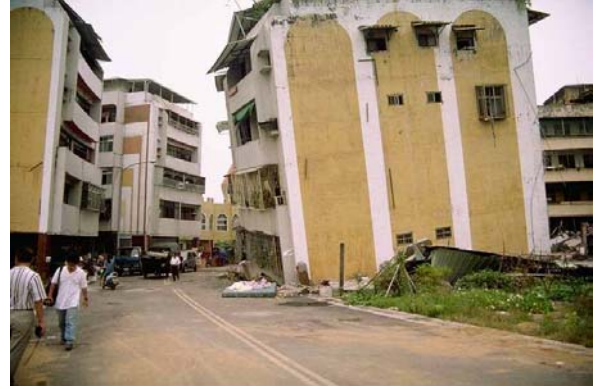
Figure 3. Collapsed 6-story reinforced concrete building on west side of Wufeng Site A (P-2 by R. Seed, 1999)
