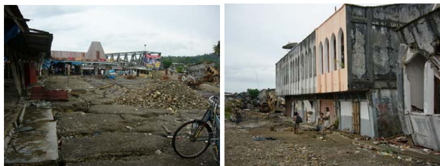
Figure 7. Effect of liquefaction and lateral spreading on RC building and truss bridge
