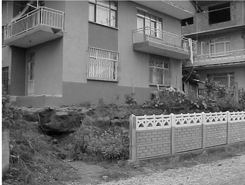
Figure 1. Two story building in Denizevler, east of Gölcük, having survived a tectonic dislocation of almost 2 meters. Observe the diversion of the fault scarp next to the building.
