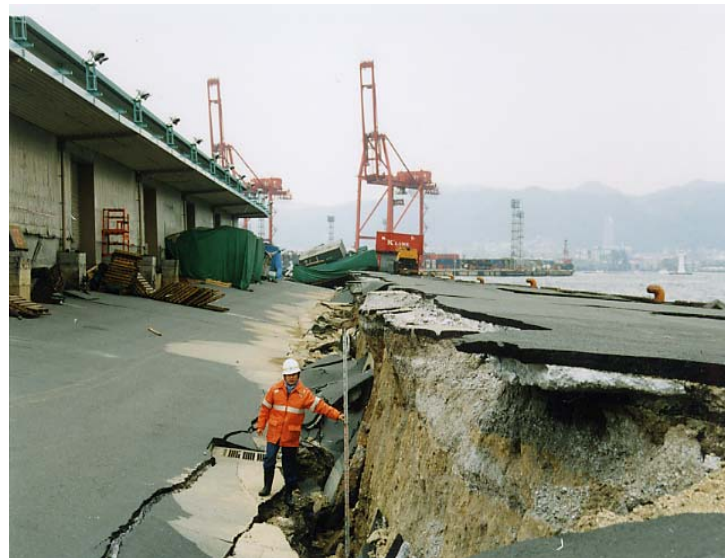
(a) Damage to a caisson quay wall at Kobe port, Japan
