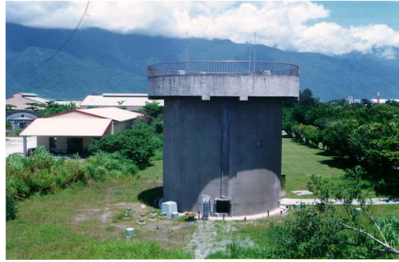
Figure 1. The 1/4 containment model at Hualien LSST
