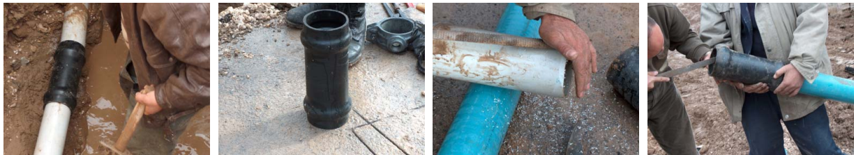
Figure 2. Repair of a PVC water distribution pipe with a PVC fitting
