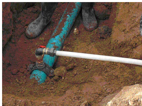
Figure 4. A new service connection to an existing PVC distribution pipe
