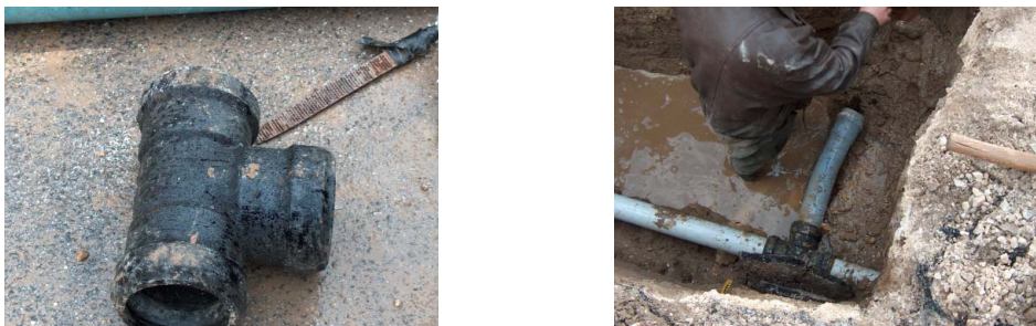
Figure 3. PVC pipe branch installation with a cast iron T-fitting
