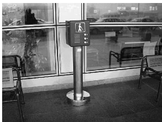
Figure 10.14. Orientation audio beacon (photograph reproduced by kind permission of Czech Blind United, Czech Republic)
