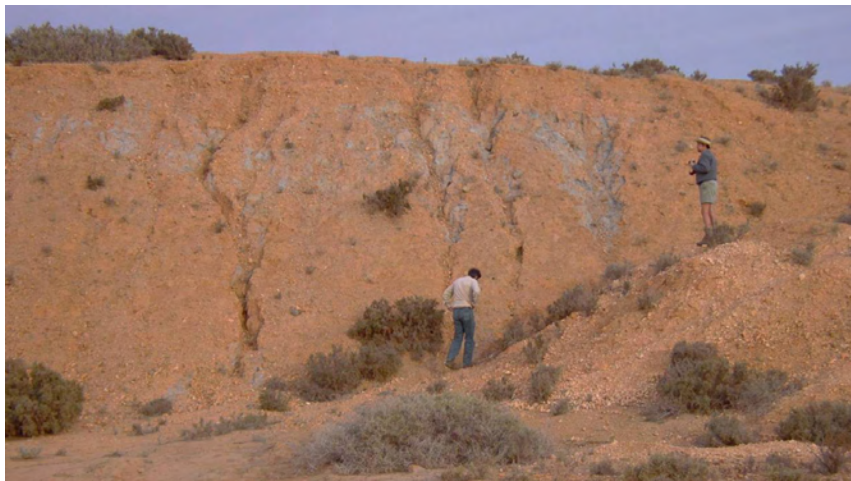
Fig.2. Rill erosion of the soil capped tailings storage facility, Radium Hill, South Australia (height of facility approximately 6 m). The soil capping is being removed, resulting in the exposure of radioactive tailings in rills.
