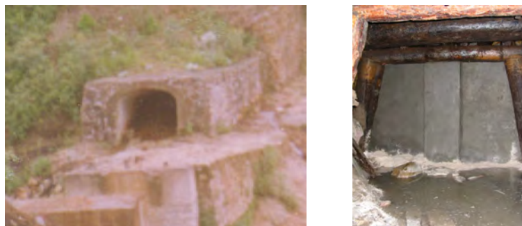
Fig.7. The inclined shaft before and during closure
