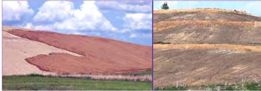
Fig.8. Covering of a stabilized waste rock pile at the mine site No. 9 in N Kazakhstan.
